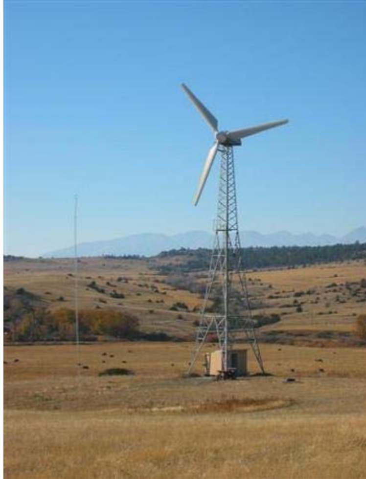
Figure 1. 65-kW Windmatic Turbine near Big Timber, MT (Source: NREL)
