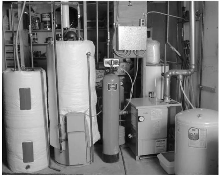
When the battery bank is fully charged, the home's second water heater (left) absorbs the heat produced by the excess wind energy. Also shown are the primary water heater, water softener, heating boiler and heating system expansion tank.
