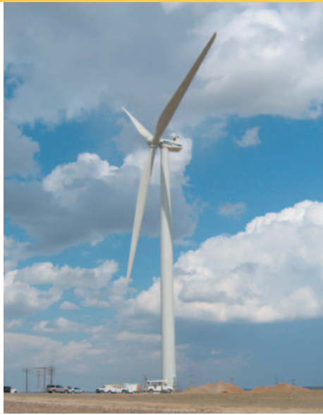
USDA provided a $1.3 million loan for this Illinois turbine.
