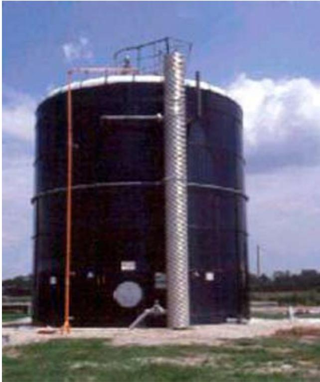
IBR digesters are designed for influent with 6 to 8 percent TS. This system will treat a medium to high OLR, between 5 to 9.1 kilograms COD per cubic meter per day (312–567 lb COD/1,000ft<sup>3</sup>/d), with a short HRT of 3 to 5 days. Systems designed to meet the NRCS Conservation Practice Standard for Anaerobic Digesters—Controlled Temperature (366) require an influent TS concentration of less than 5 percent and a HRT of 1 to 6 days.
