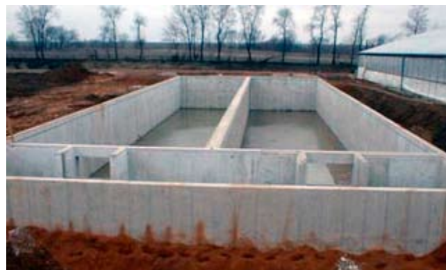
Figure 7 Parallel plug-flow digester cells under construction prior to cover installation
