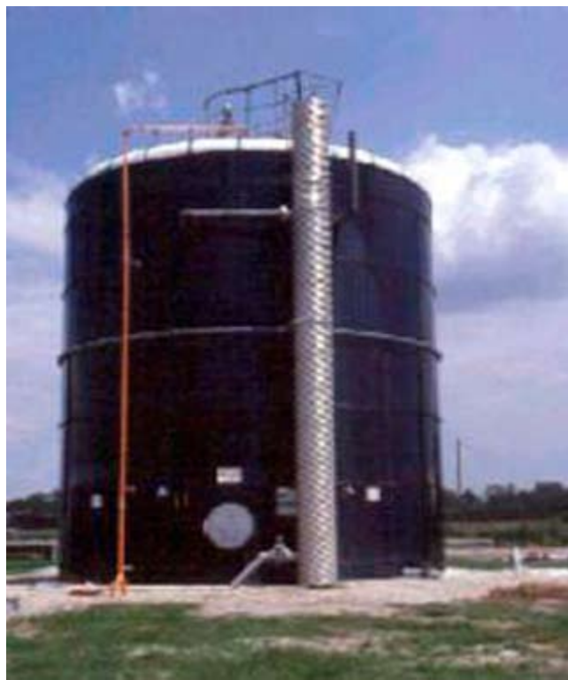
Figure 9 Fixed-film digester
