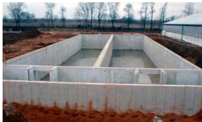
Mixed digesters can process manure over a wide range of TS. Continually stirred tank reactors used for manure digestion typically have OLRs between 1 to 10 kilograms COD per cubic meter per day (62–32 lb COD/1,000 ft<sup>3</sup>/d). The HRT of these systems treating manure is typically between 5 to 20 days. The NRCS Conservation Practice Standard for Anaerobic Digesters—Controlled Temperature requires an HRT of 17 days for mixed digester systems.
