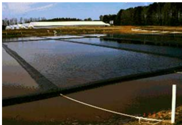
Figure 6 Partially covered anaerobic swine lagoon
