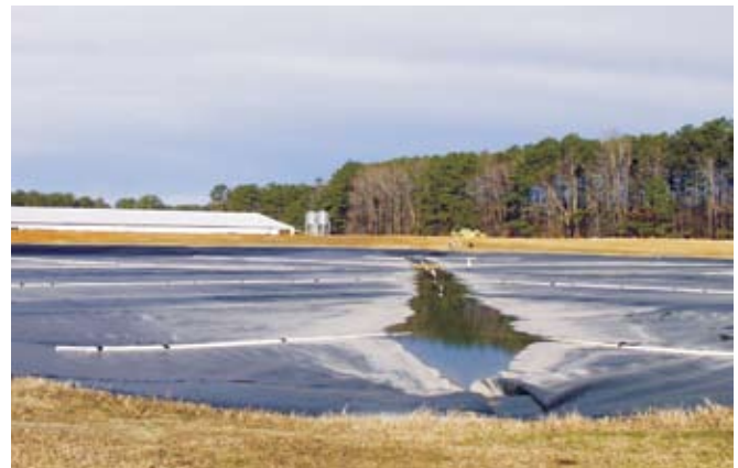
Figure 1. Ambient-temperature covered digester at 4000 sow farrow-to-wean farm in Johnston County, N.C. Cover was installed in 1998.
